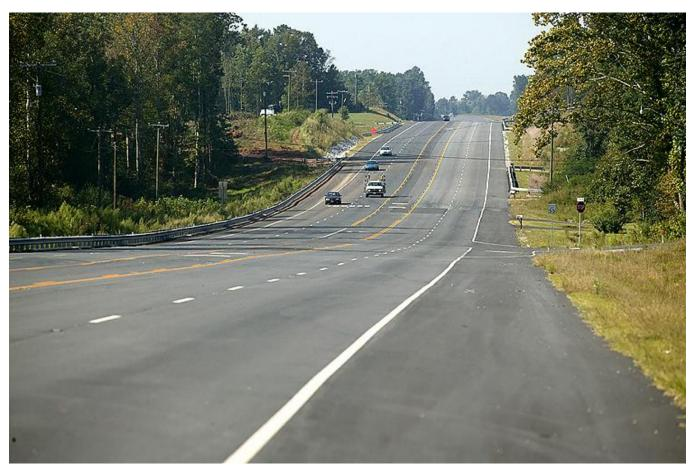
A five-lane paved section can provide a big capacity boost and improvement in Level of Service, but is vulnerable to capacity degradation by frequent points of access, visible in this image of recently improved US 58 in Virginia.
