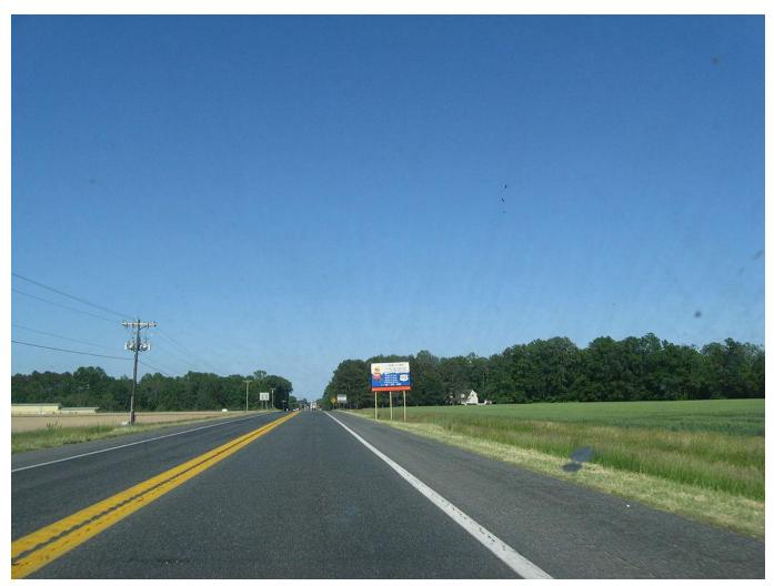
The Low Build option would optimize 2-lane capacity by easing grades and restricting access points and driveways, as on this improved section of Route 113 near Newark, Delaware.
