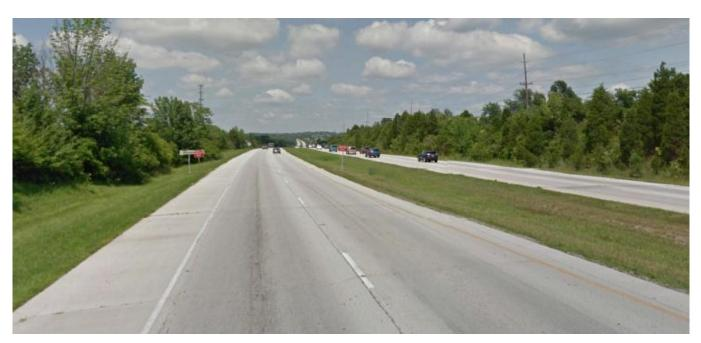
The four-lane section with grass median concept typically uses "open" drainage and provides physical and visual separation of opposing directions of traffic; this example is SR 48 in Warren County, looking north toward Lebanon
