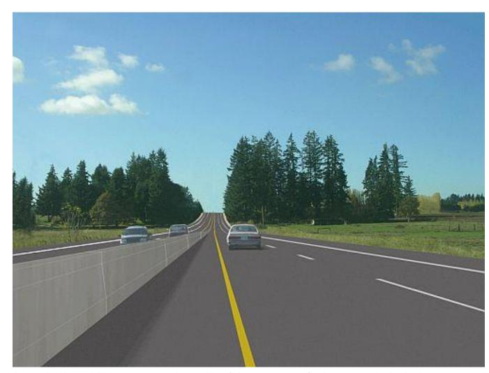
The paved median with barrier concept provides a stable, safe long-term strategy for the SR 63 corridor, but has limitations in turn movements and requires a high degree of access management, as shown in this illustration of proposed improvements to State Route 502 in Battle Ground, Washington
